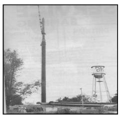
Every day the water tower structure gets higher, higher and higher. Pittsburgh Des Moines Steel Co. has the contract for the construction of the 300,000 toro spherical water tank at a total cost of \$209,300. The job is to be completed late this summer. The present 25,000 gallon water tower is expected to be torn down when the new one is put into operation. Reprinted from The Big Creek News, June 3 1976.
